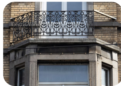
Garde-corps de balcon
